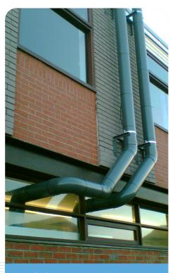
Harmful fumes are extracted to atmosphere via PVC ductwork
